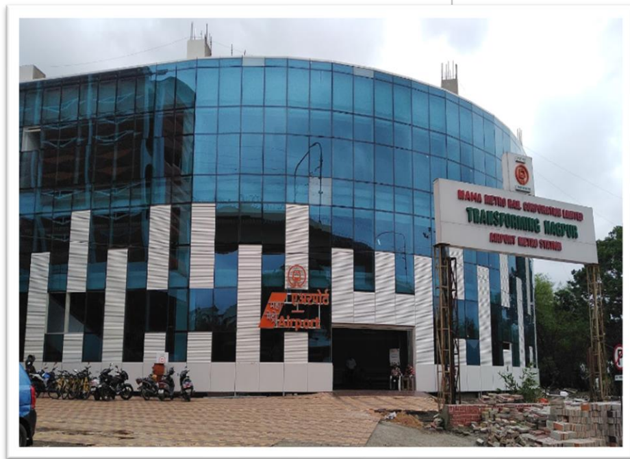
MAIN ENTRANCE OF AIRPORT METRO STATION
